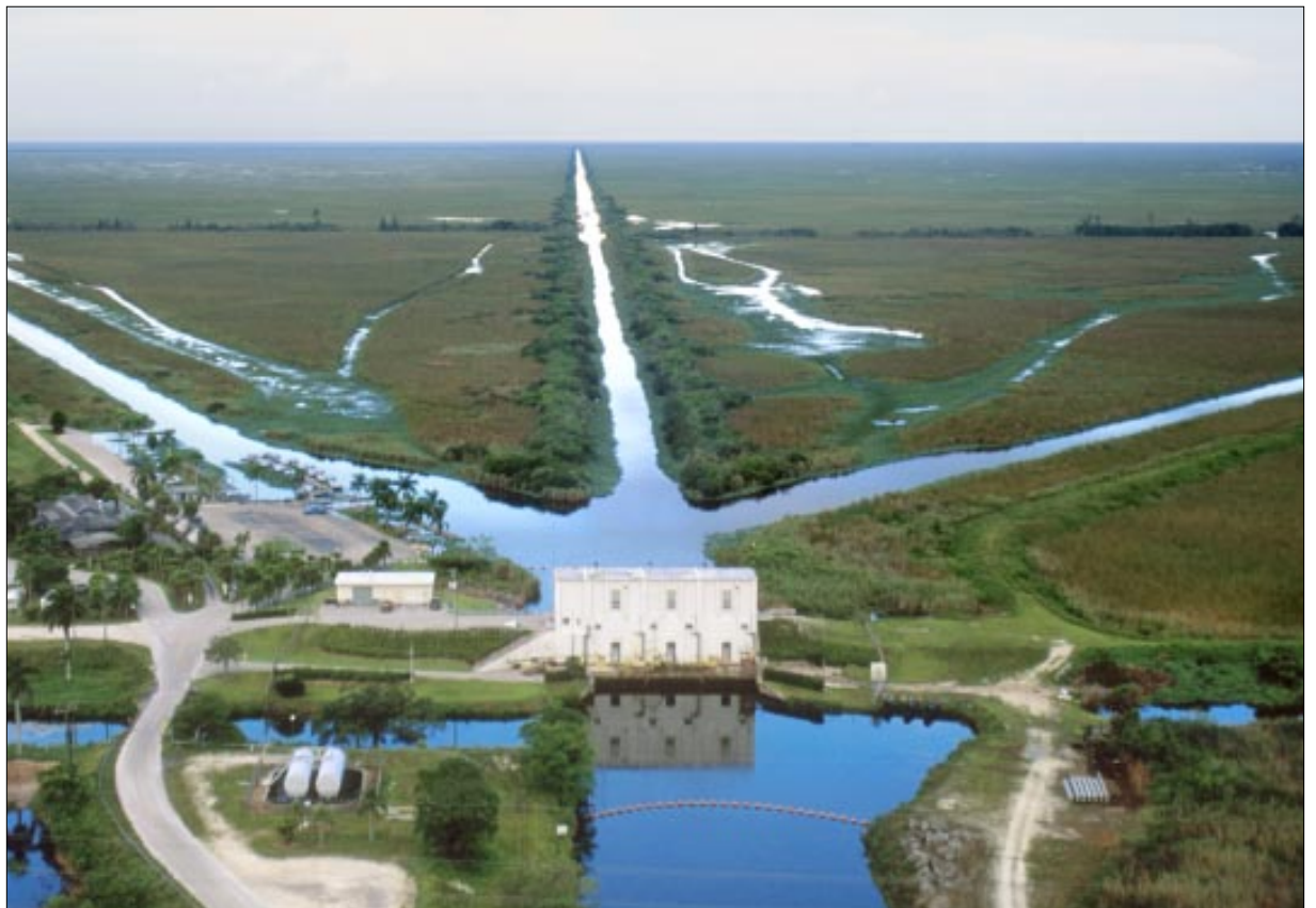
The S-9 pumping station, located in Broward County, is the primary discharge structure for the C-11 West Basin, one of the urban tributary basins discharging stormwater runoff into the Everglades Protection Area.
